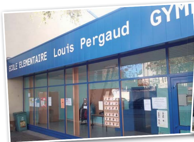
Bardage Gymnase Louis Pergaud
